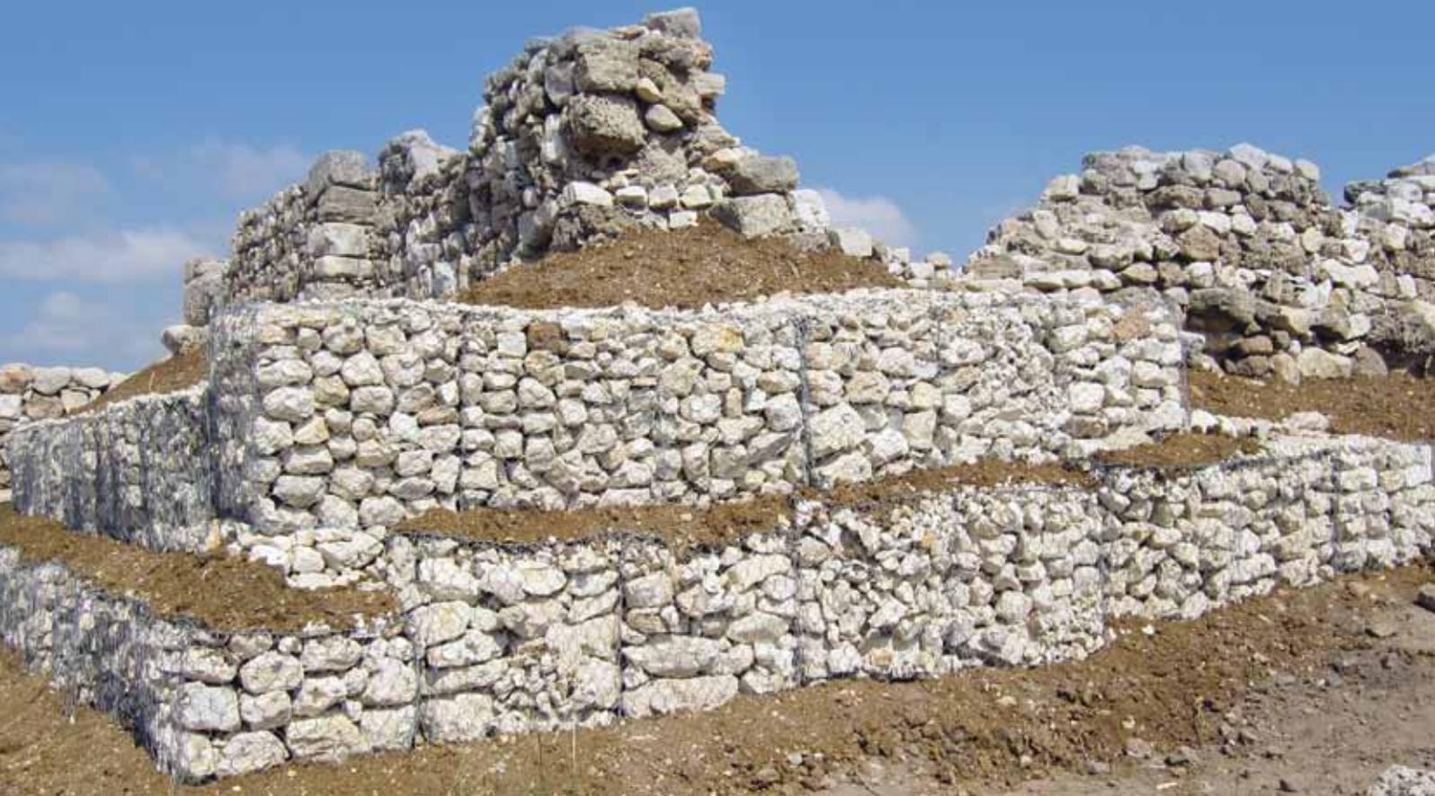
2. *At the southern side of the Great Residence, also dating to the Bronze Age period, an old reconstructed stone wall had partially collapsed due to the feeble retaining wall. The latter wall was rebuilt according to the traditional method.*
