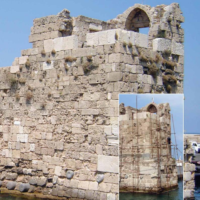
The northern Medieval tower presented critical under water structural damages mainly at the southeastern corner foundation.
